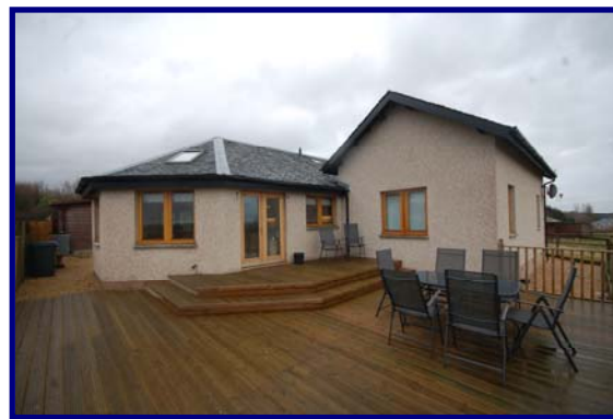
South West Elevations – Kitchen extension on left and bedroom extension on right
