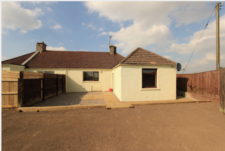
Southern elevation of house from rear garden
