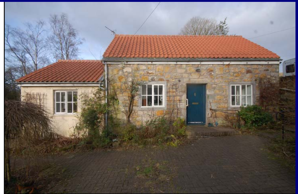
South elevation of cottage
