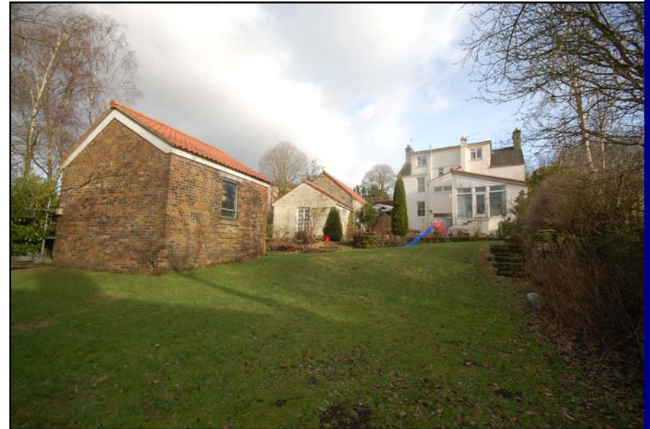
Shed on left, cottage in middle, house on right
