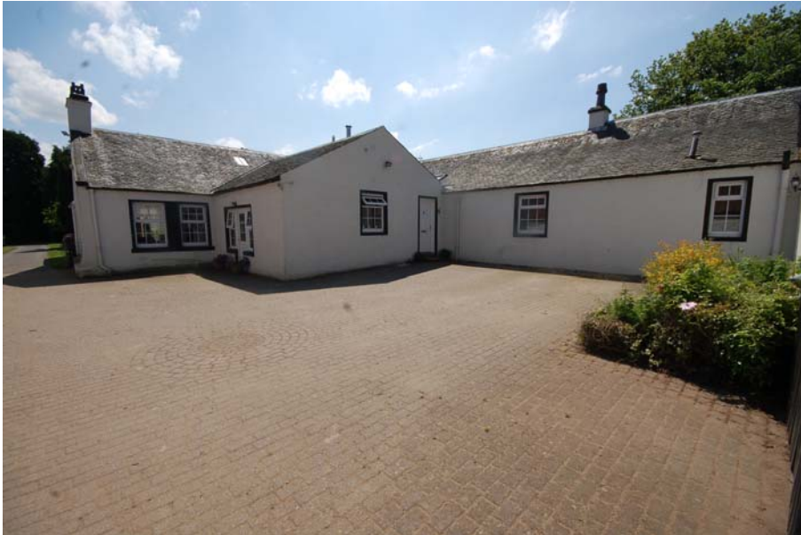
North and East elevation of the house
