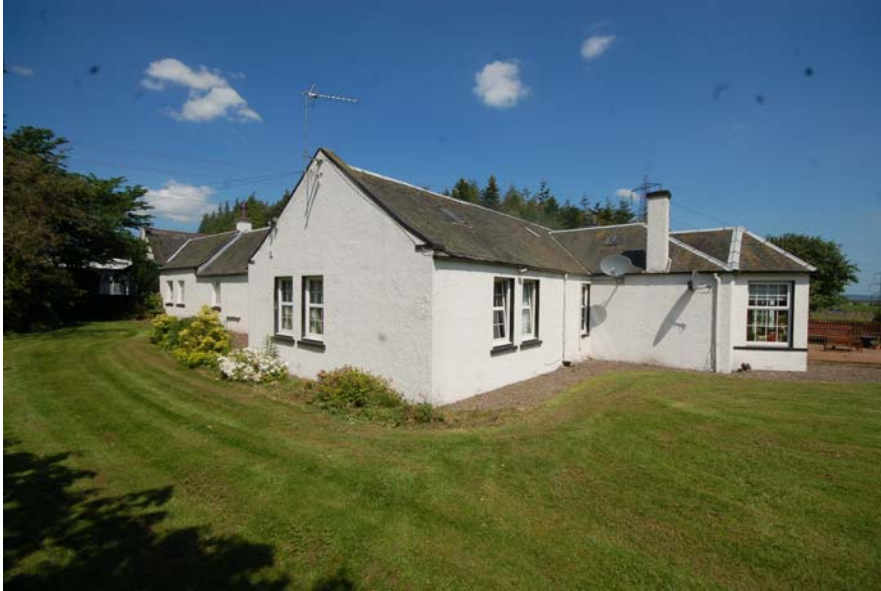
West and south elevation of the house
