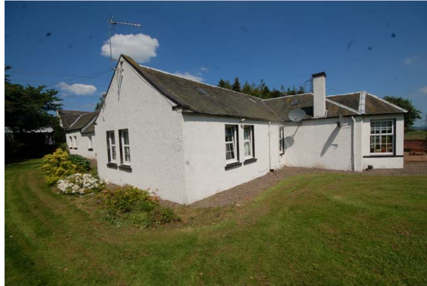
South and west elevations of the house
