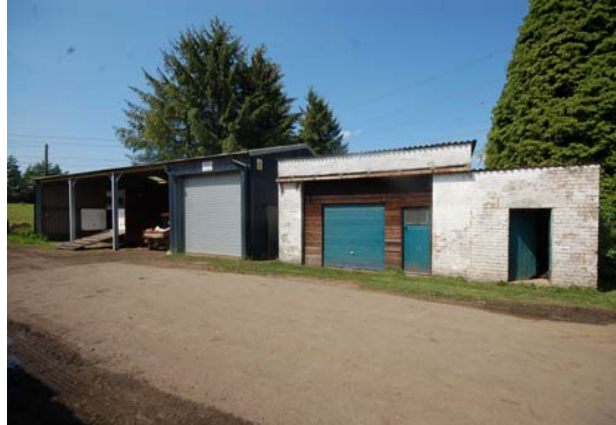
Portal Framed Shed (Lot 2)
