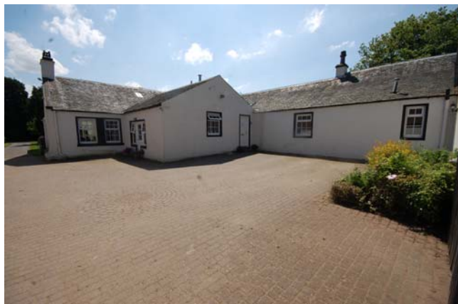
North and East elevation of the house
